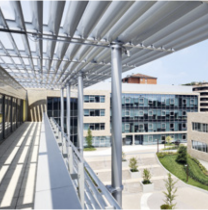
ALB fisse, pensilina ALB-passive, cantilevered
